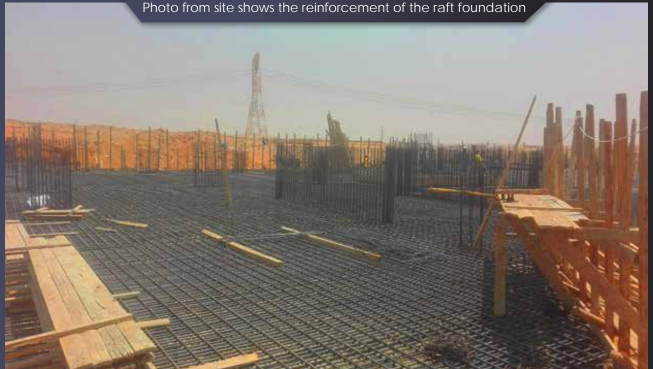
Photo from site shows the reinforcement of the raft foundation
